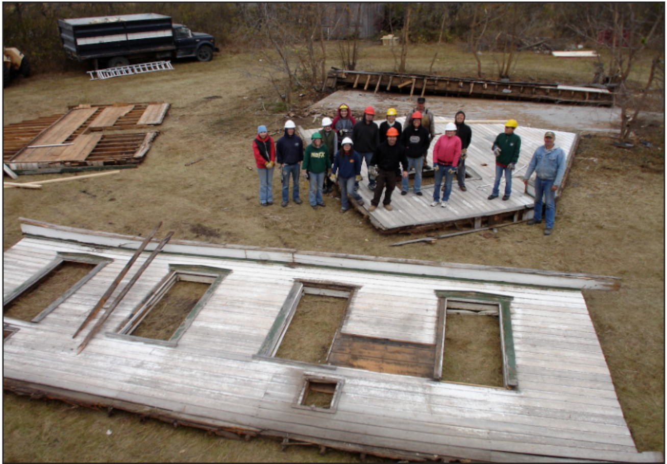
Figure 1: The deconstruction of the Crystal River Schoolhouse.
